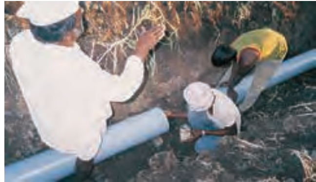
Installation of Supreme pipeline in the field
